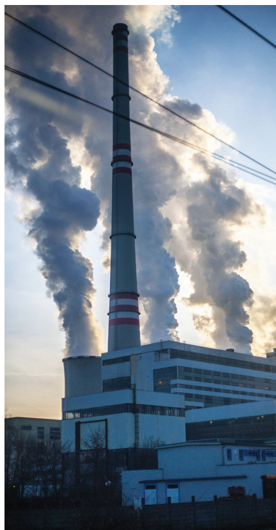
Chvaltice coal-fired power plant, Czech Republic. PHOTO: Laura Otýpková, Frank Bold
